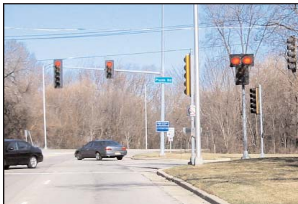
Figure 3-10. Supplemental Signal for an Intersection in the Middle of a Reverse Curve.
