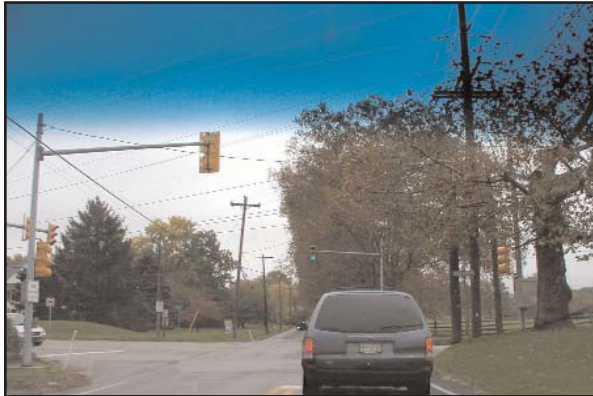
Figure 3–2. Post-Mounted Signal Blocked by Vehicle.
