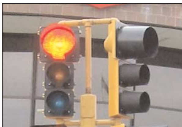
Figure 3-11. Comparison of Signal Heads Using 8-in. and 12-in. Lenses.
